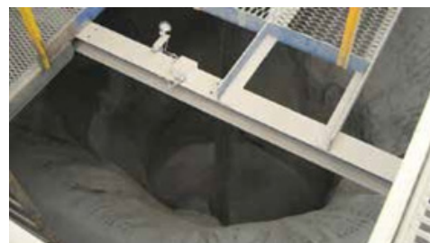
Rathole: The centre portion of the bin empties first in the form of a funnel.
