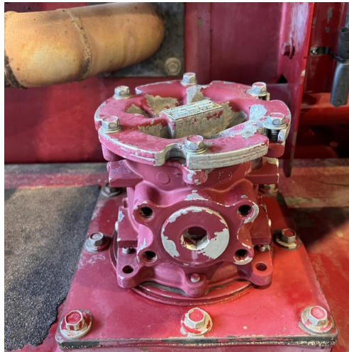
Figure 2: OEM hydraulic filter housing with the OEI Filter cap installed.
